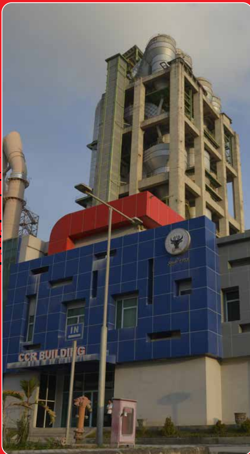
CCR Building Indarung VI
